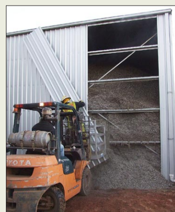
REPAIR work continues at the damaged shed.
